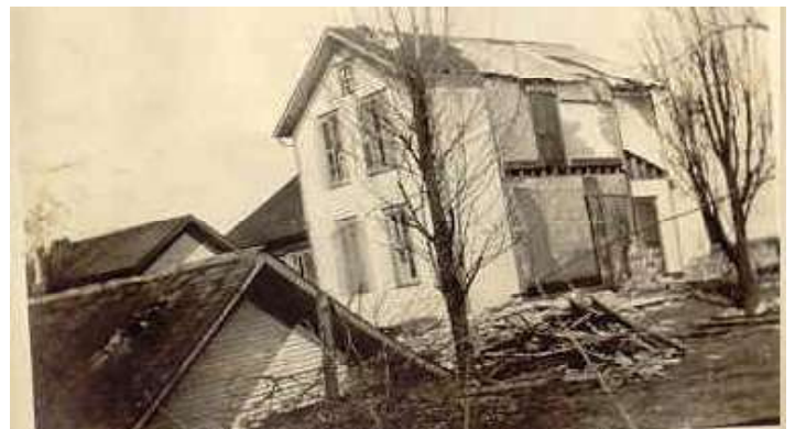
Another view showing the total destruction of the town of Brunersburg in 1920.
